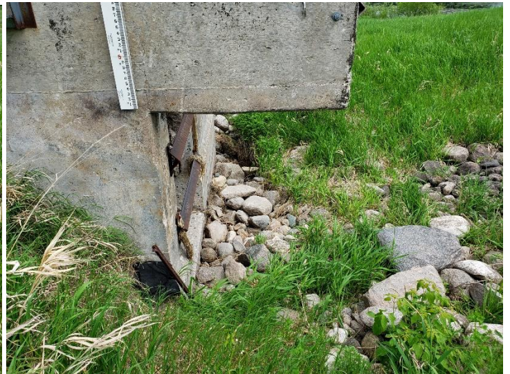
South side, looking east
