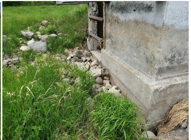
South side, looking west
