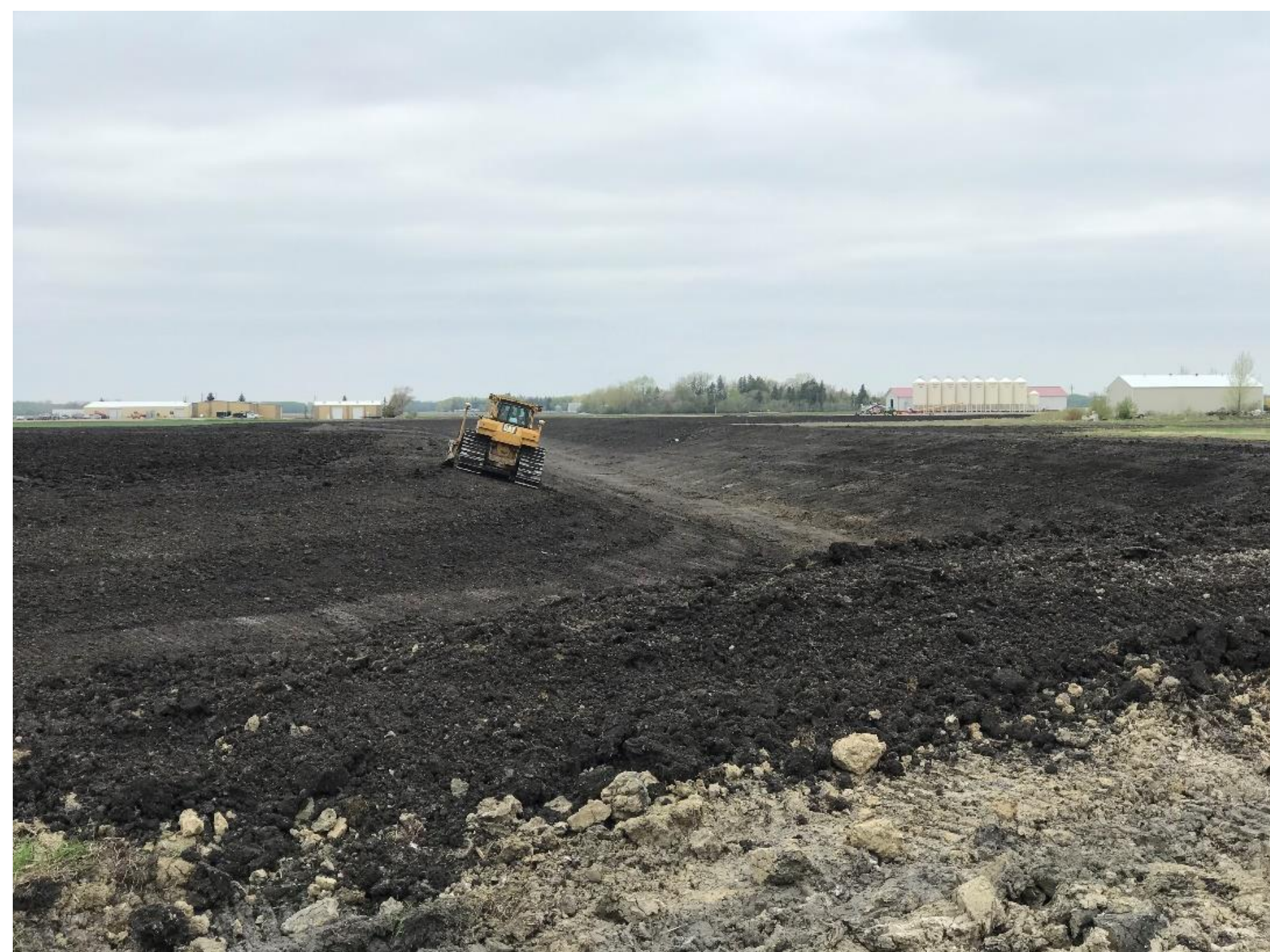
Photograph of diversion construction at the north end of the project area on May 20, 2020. Photograph courtesy of Robert Sip.
