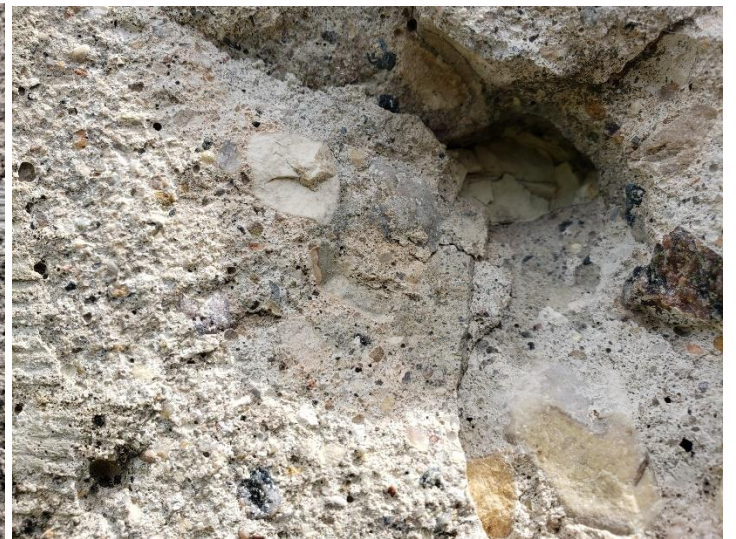
Spall, probably due to chert rock
