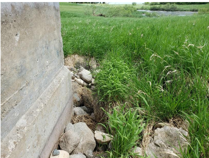
South side, looking east
