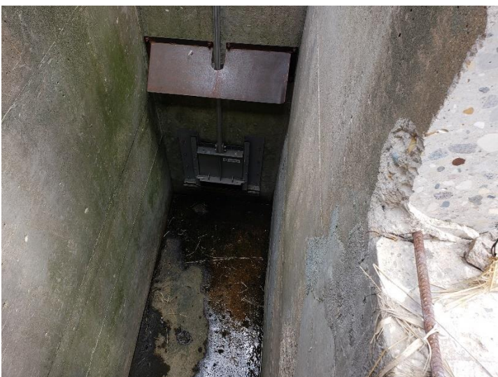
Gate, need nuts tightened
