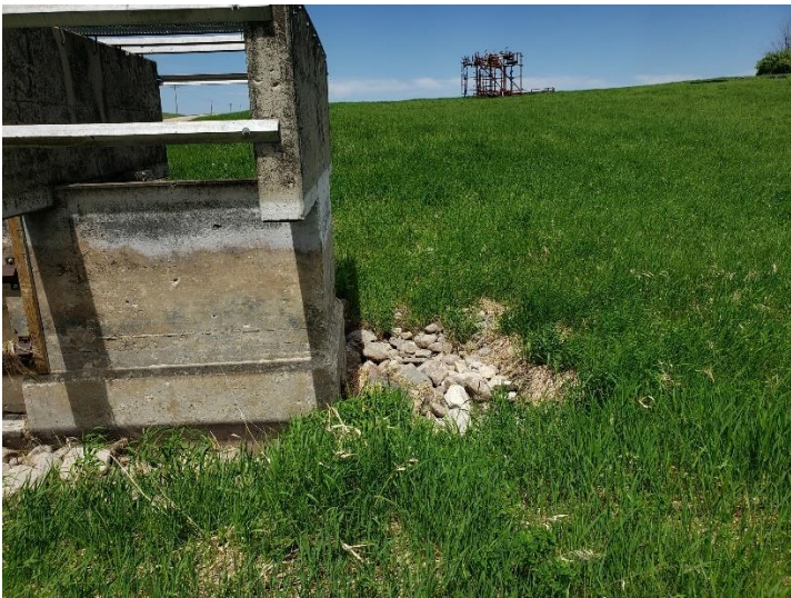
East side, settlement of ground next to structure
