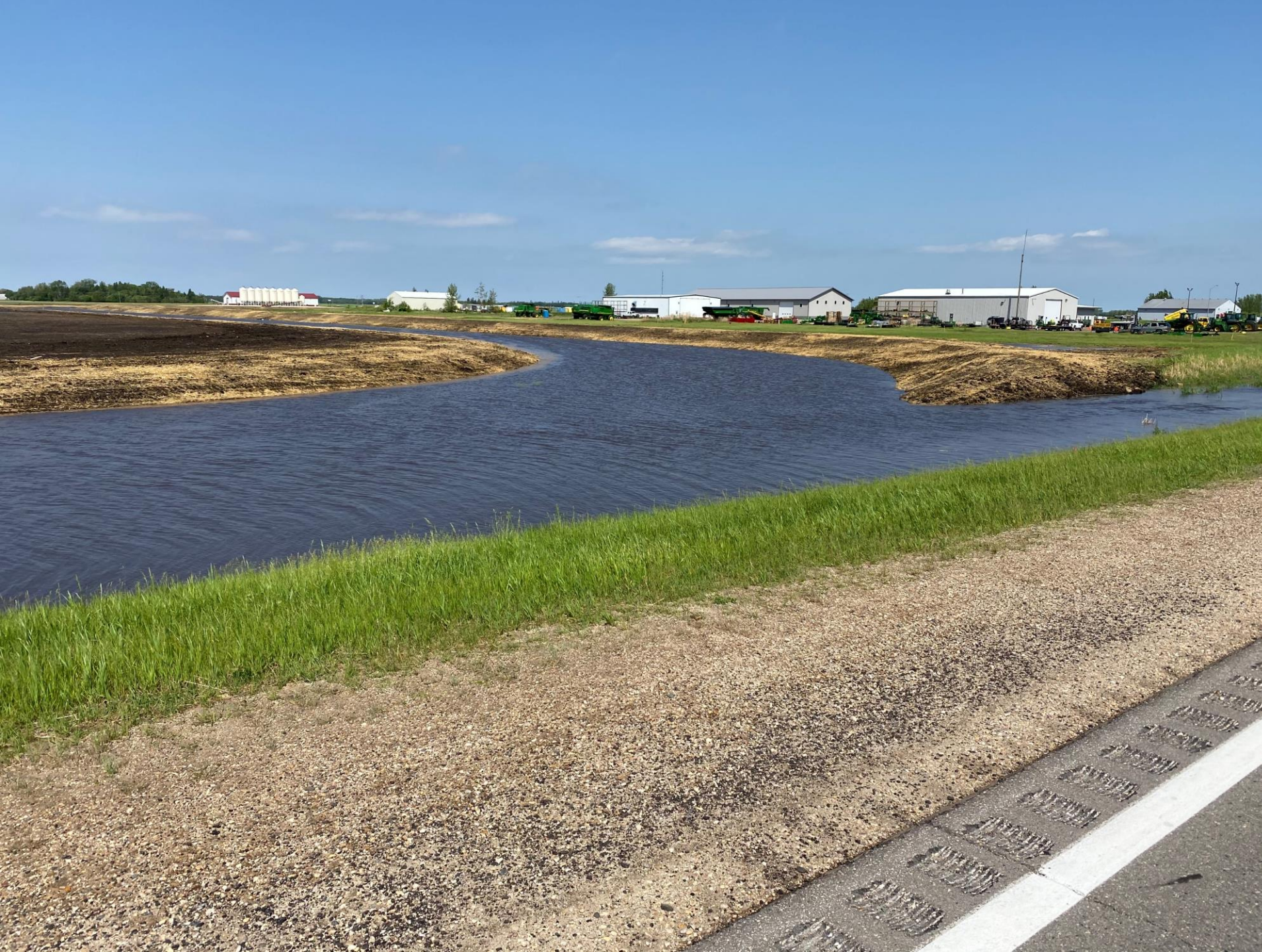
Photograph of diversion construction at the north end of the project area June 9, 2020. Photograph courtesy of Myron Jesme
