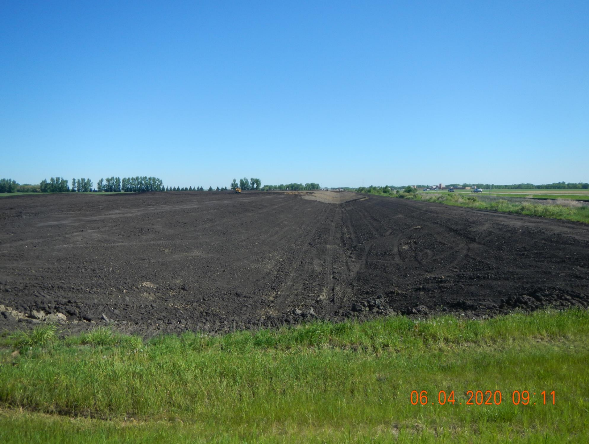
Photograph of diversion channel construction looking north from CSAH 7 and parallel to State Highway 32. South end of the project area on June 4, 2020. Photograph courtesy of Myron Jesme
