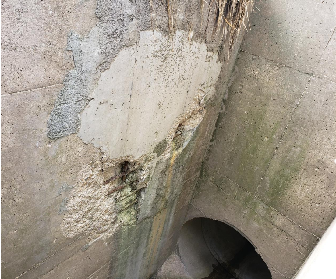
South wall, patch with additional concrete loss
