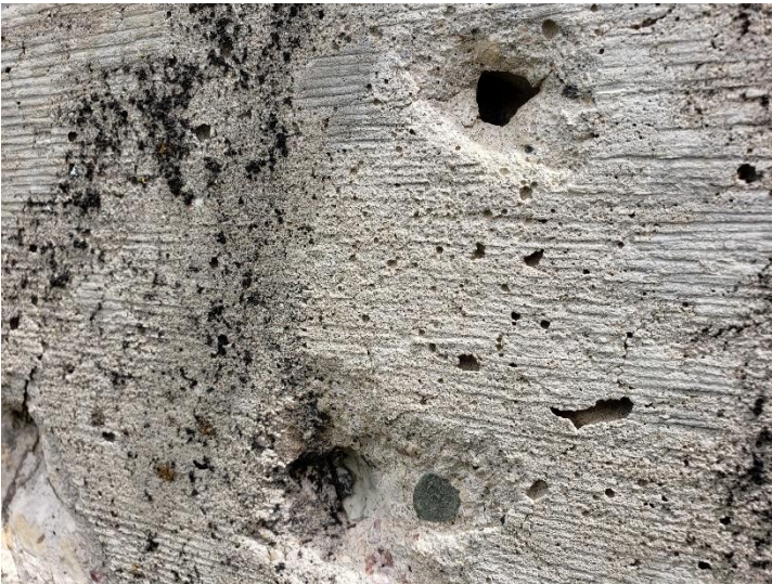
Close up of spall area
