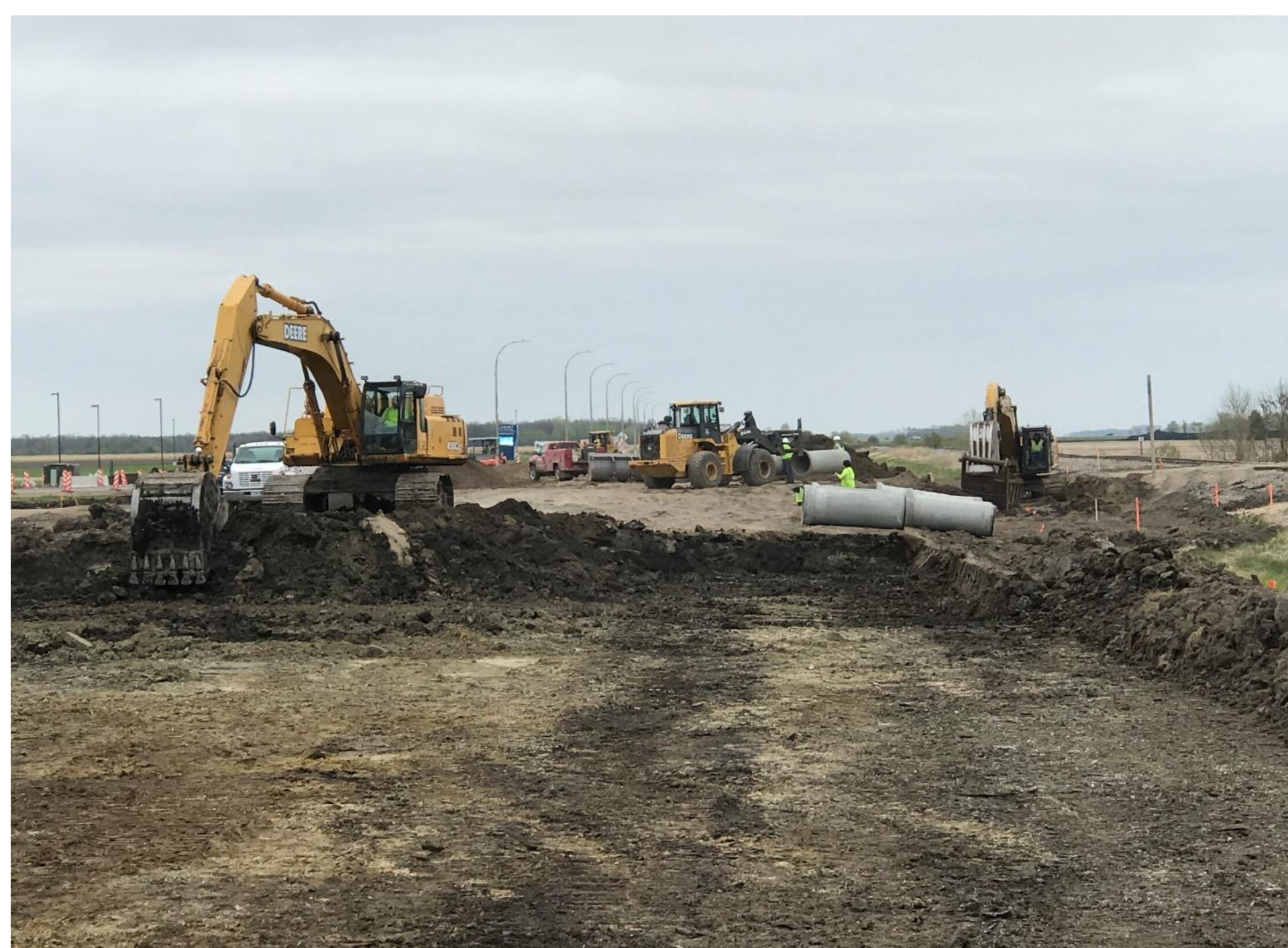
Photograph of a new roundabout being installed on State Highway 32 on the south end of the project area on May 20, 2020. Photograph courtesy of Robert Sip.
