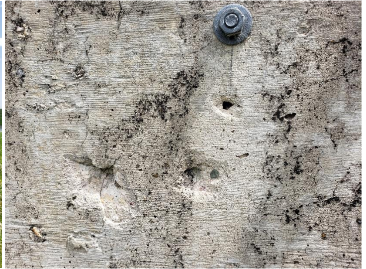
Spall on north end of west wall
