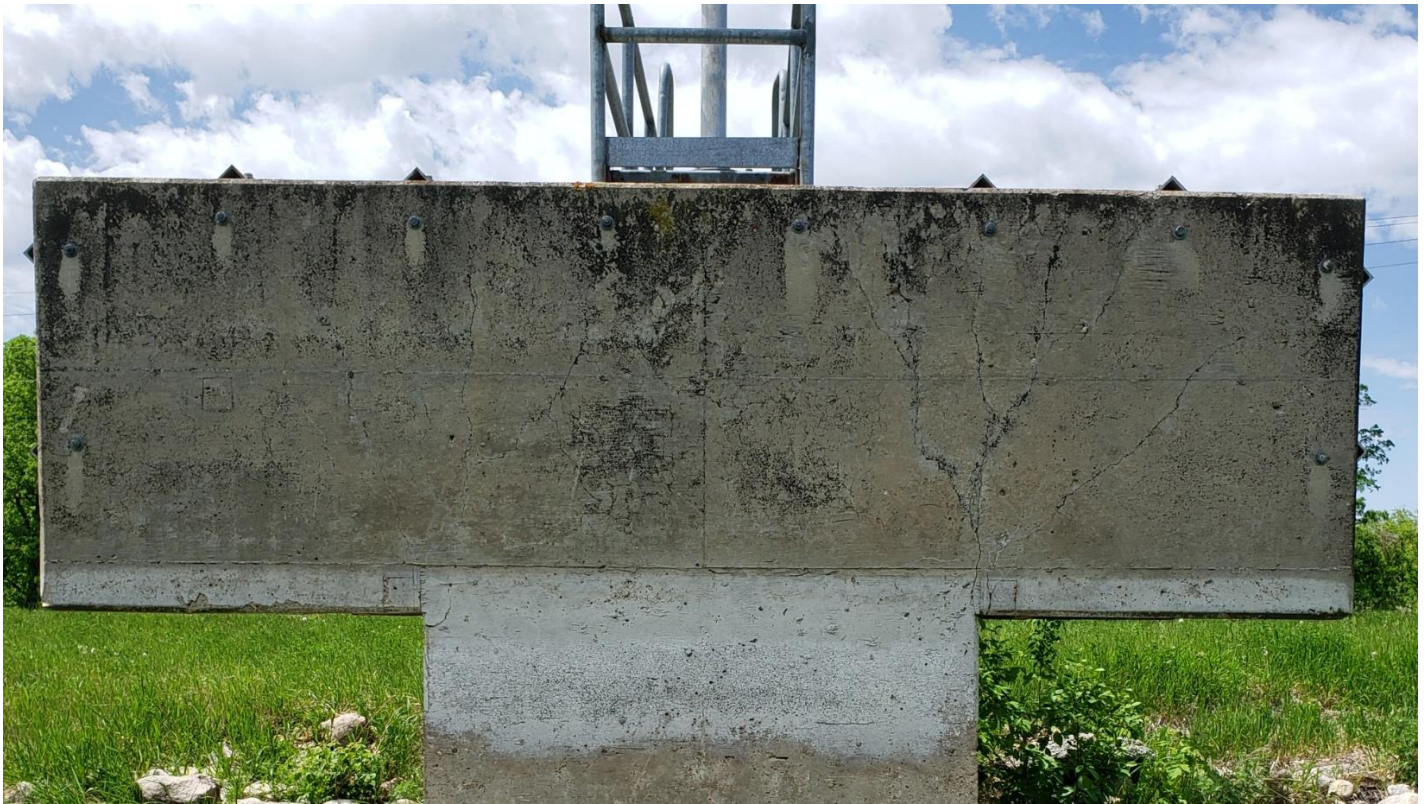
Cracking in upper portion of wall, radiating out of cantilevered corner
