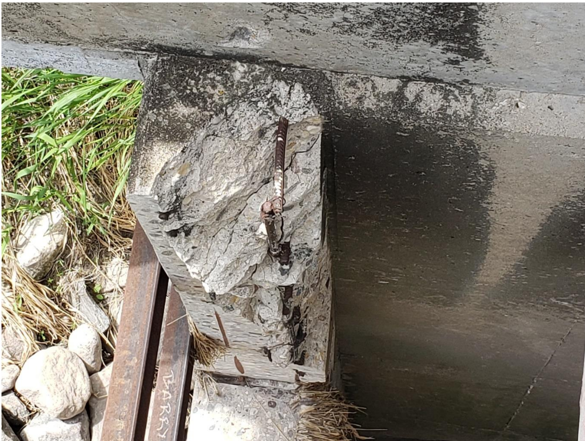
Crack in wall from cut out
