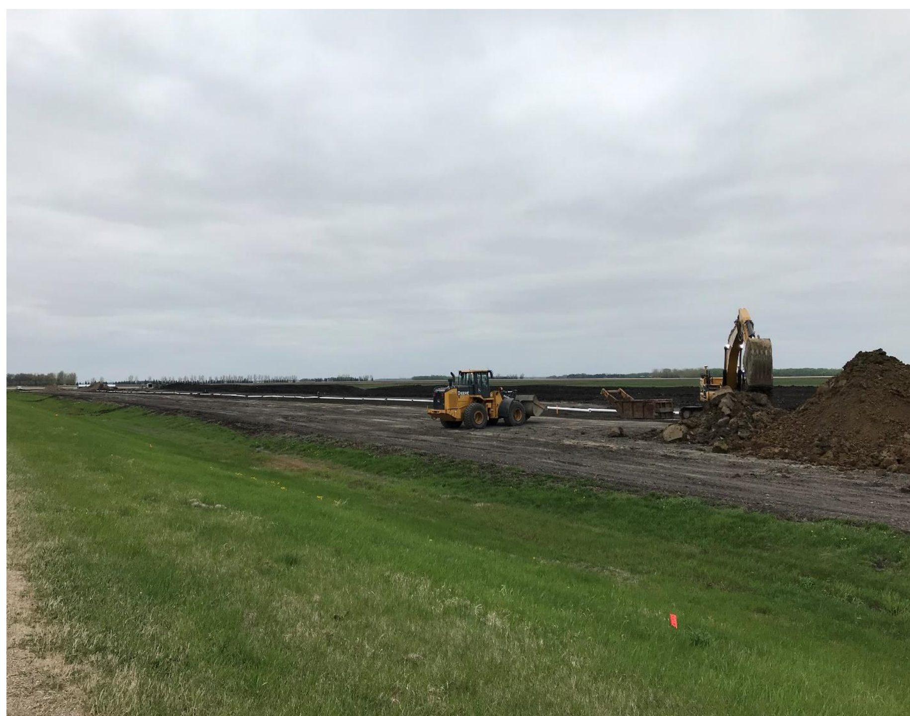
Photograph of new steel pipe being installed on State Highway 32 on the south end of the project area on May 20, 2020. Photograph courtesy of Robert Sip.
