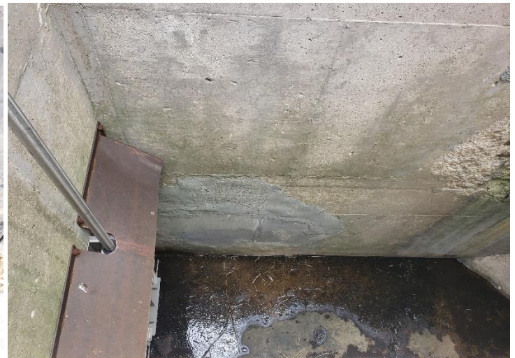
Patch, south wall
