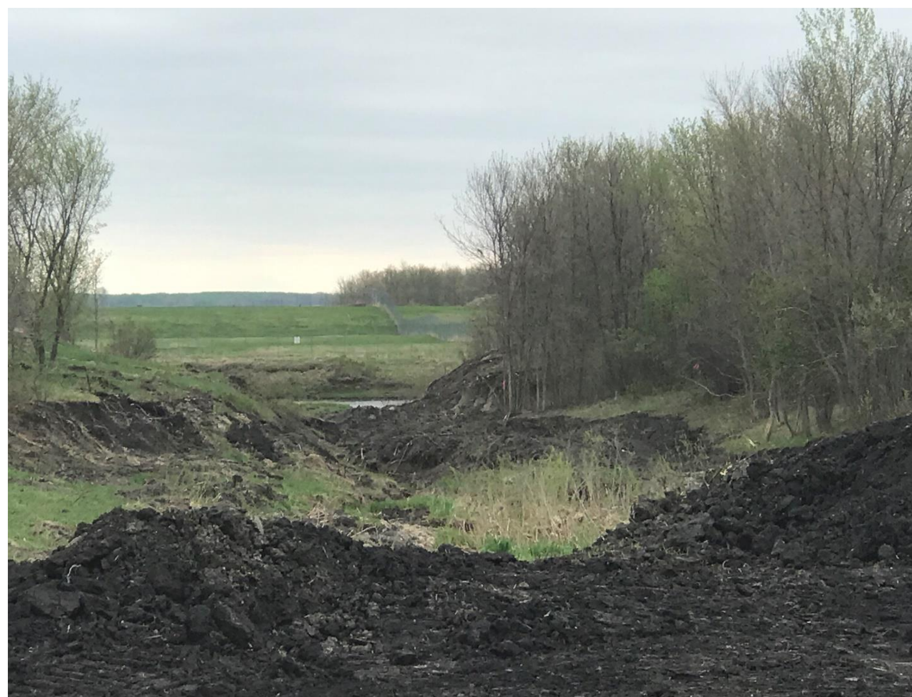
Photograph of the existing outlet channel into the Red Lake River that is currently under construction on May 20, 2020. Photograph courtesy of Robert Sip.
